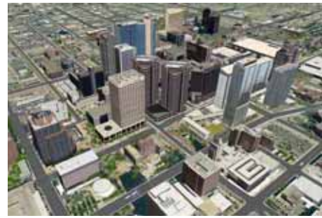
Digital Phoenix Project
